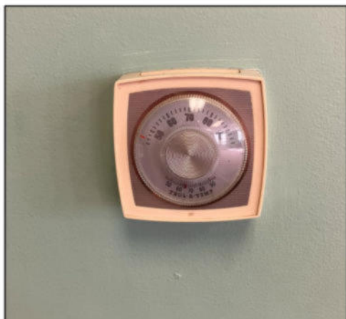
Existing manual analog thermostats
