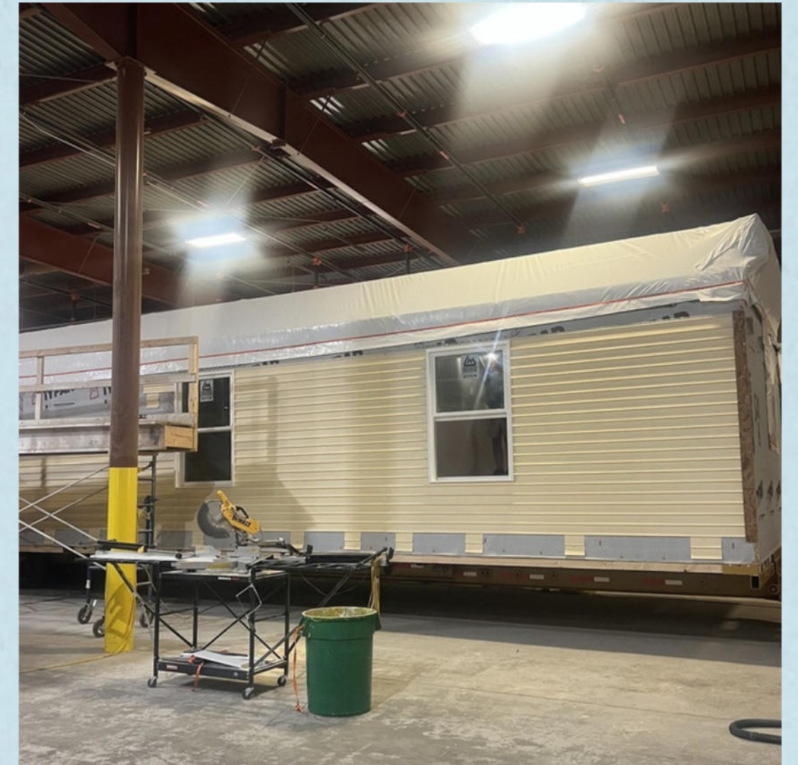
Modular housing construction at Preferred Building Systems in Claremont, NH
