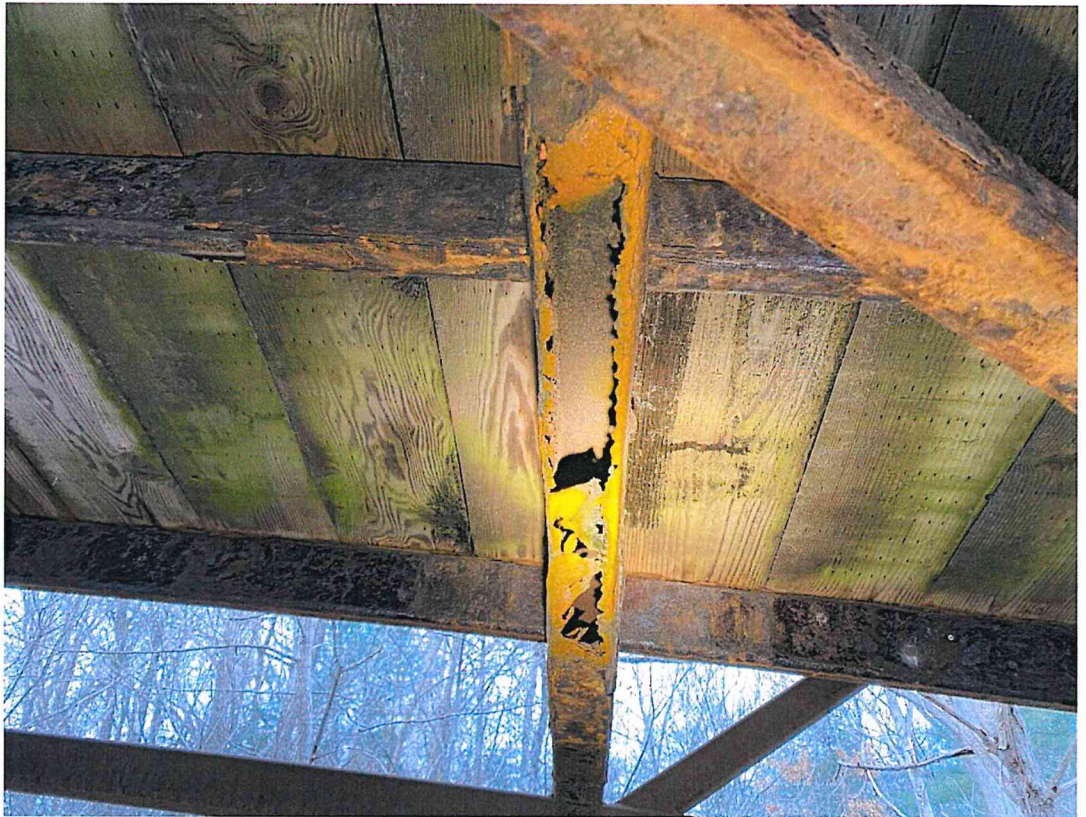
Bottom of Floor Beam 6 on upstream end.
