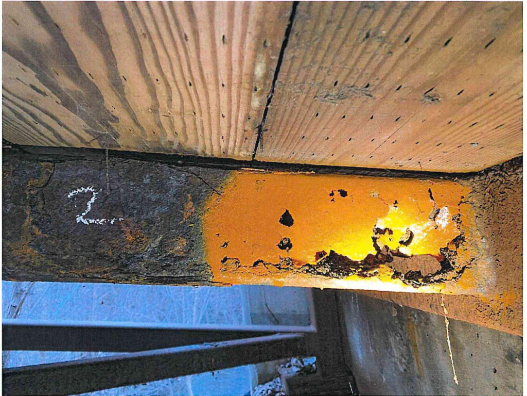
End of Stringer 2 at Floor beam 7 connec on. Downstream Side.
