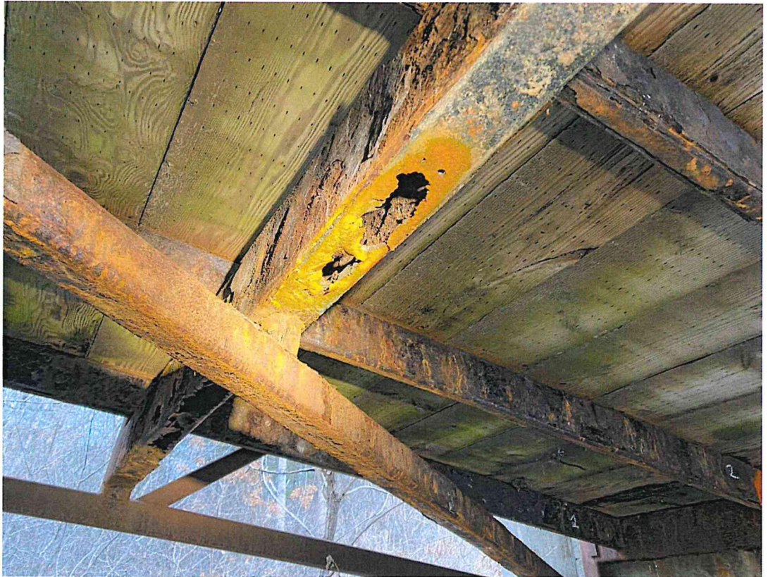
Bottom of Floor Beam 6 in center section.
