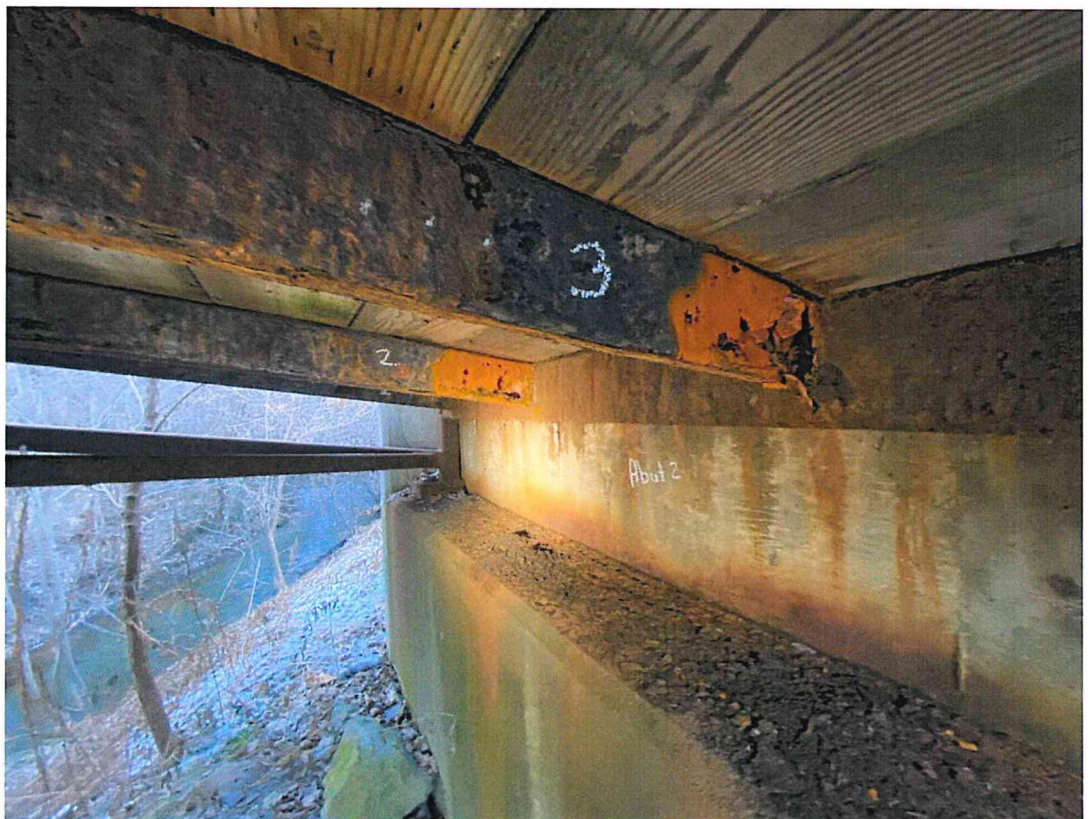
Large Holes in Abutment 2 end of stringers 2 and 3 near connection to Floor Beam 7.
