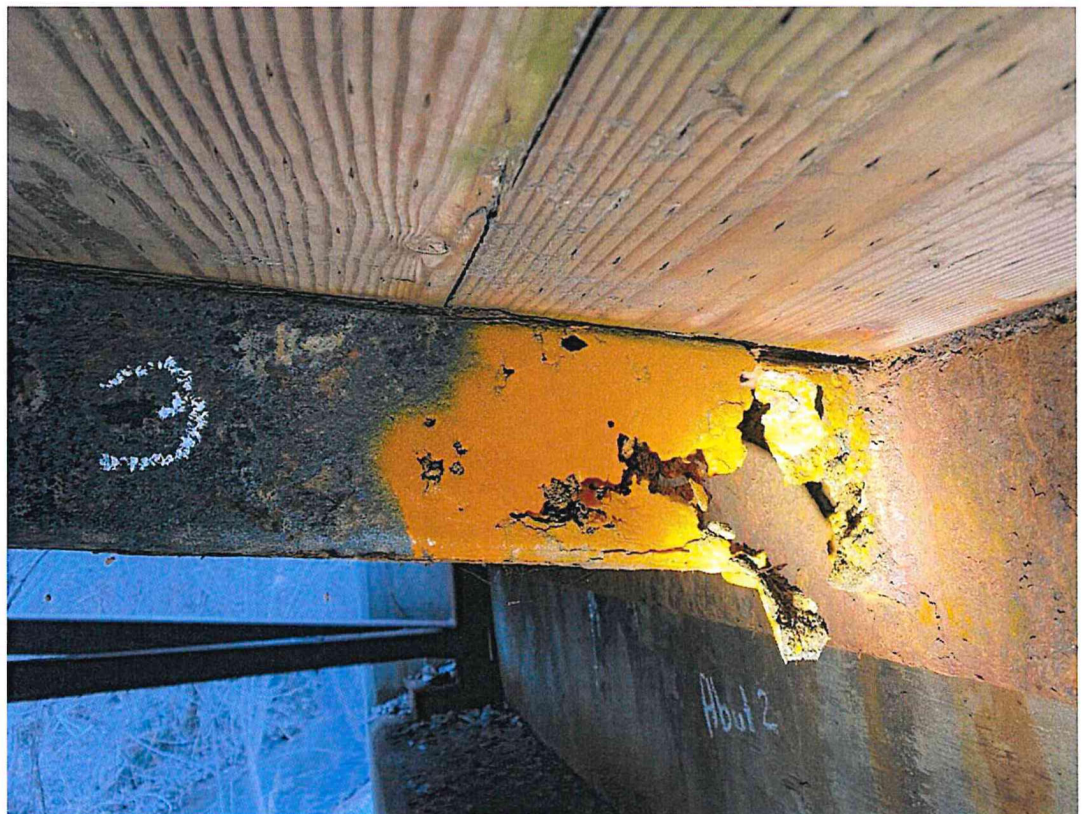
End of Stringer 3 at Floor beam 7 connec on. Downstream Side.
