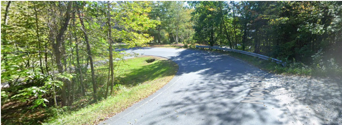
Bottom Left Hairpin With Expose Guardrail
