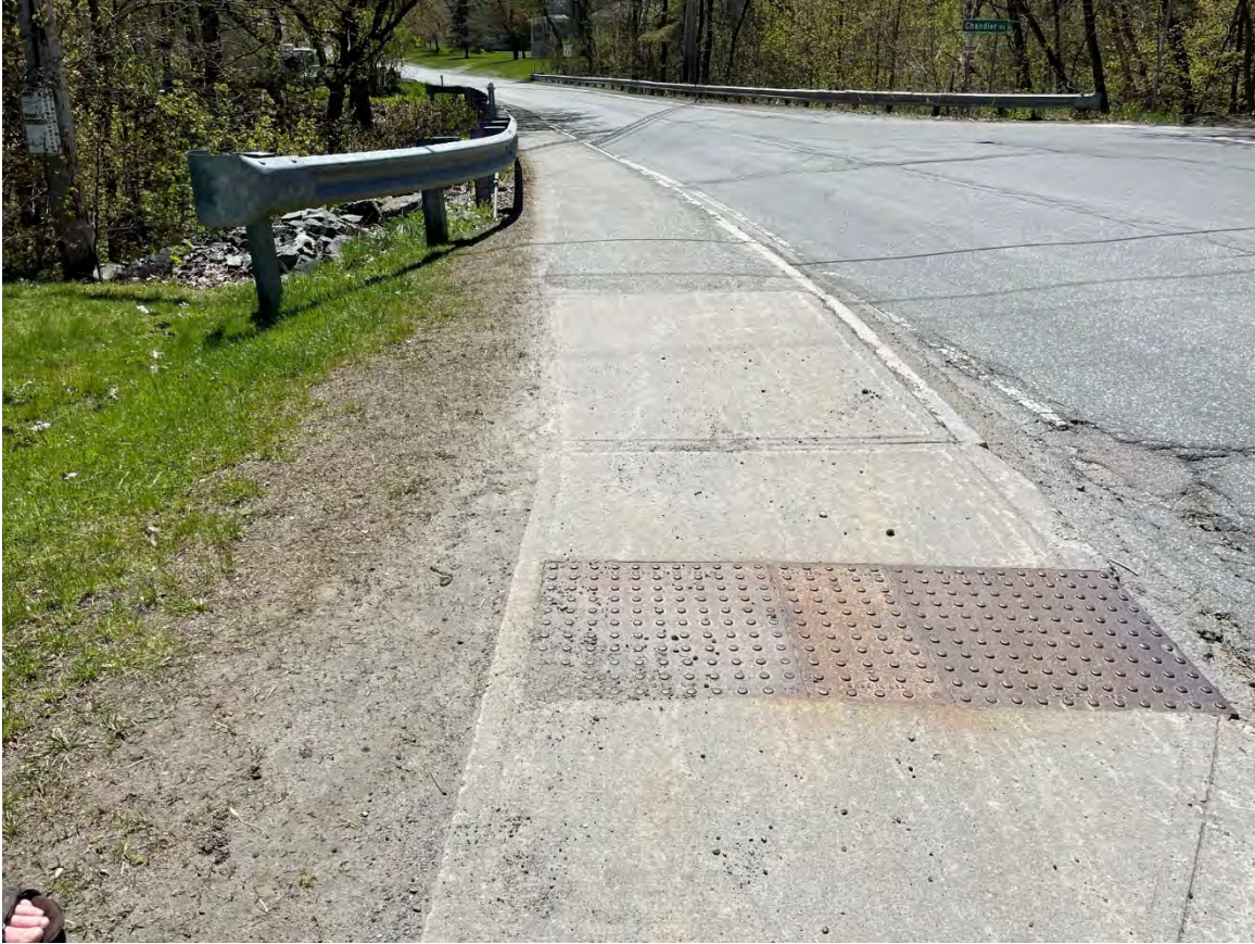
End of sidewalk segment at A Street.
