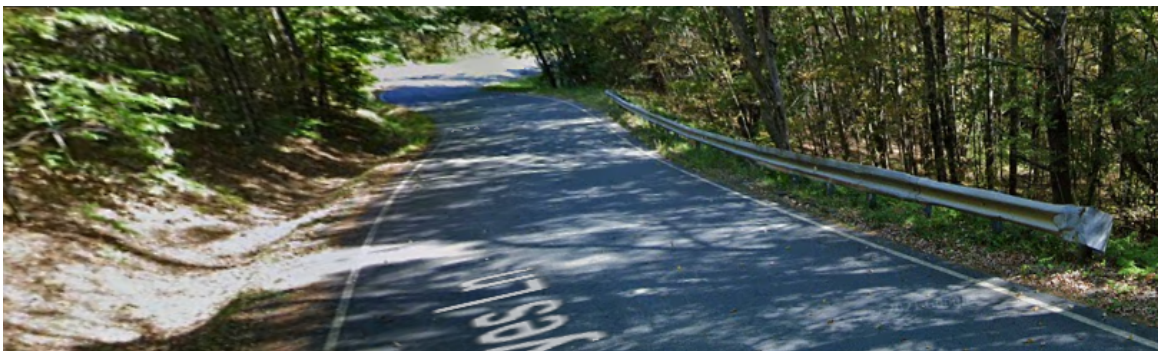
Bottom Straight Guardrail
