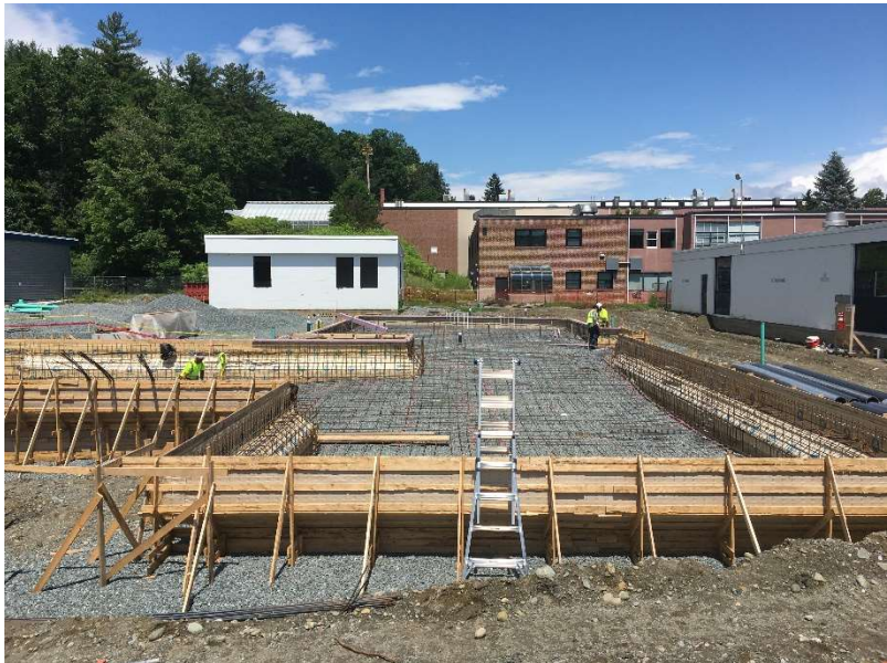
Formation of Pool Shell and Steel Work
