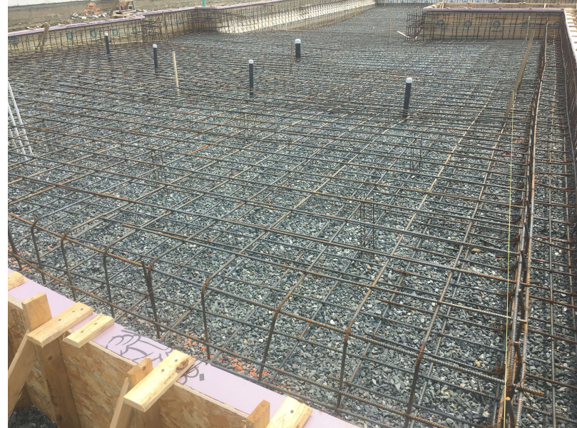
Formation of Pool Shell and Steel Work
