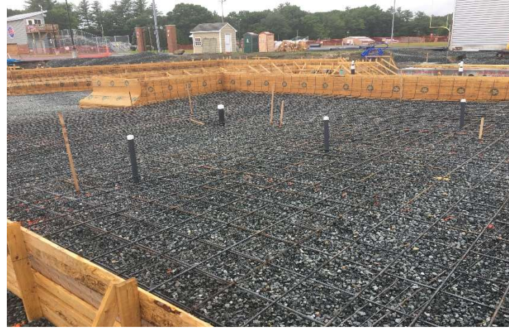
Formation of Pool Shell and Steel Work
