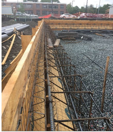
Formation of Pool Shell and Steel Work
