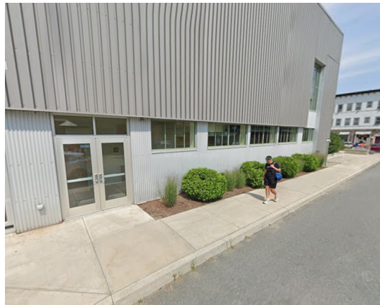
View of 76 Gates from Common ROW:
