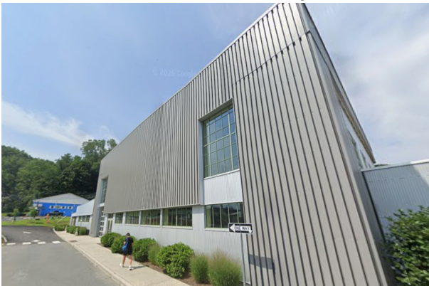
View of 76 Gates from Rear of Filling Station
