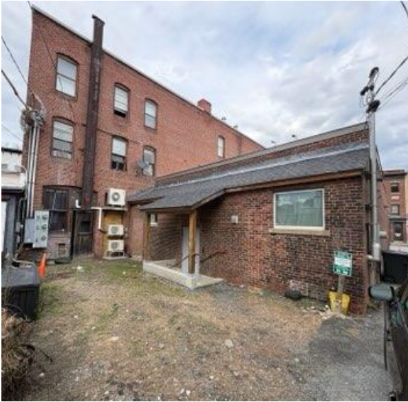
Rear of 60 Gates & 79 S Main
