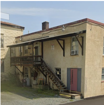
View of 93 S. Main Facade
