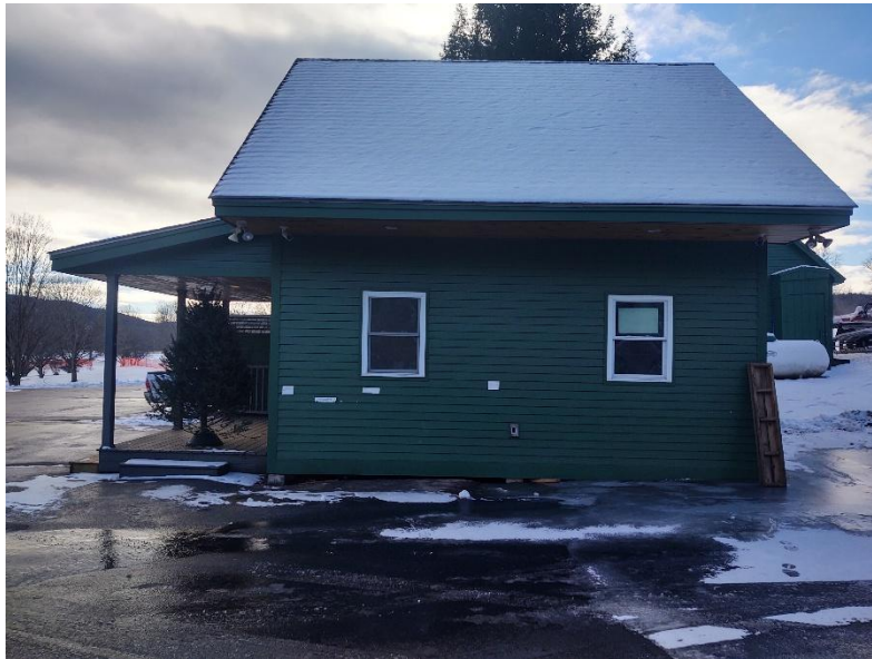
Side view of building to be removed.
