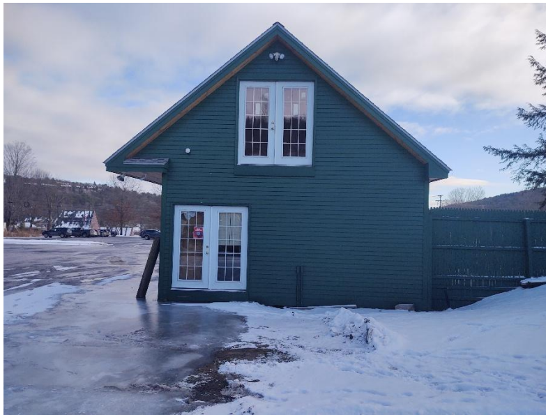
Rear view of building to be removed.
