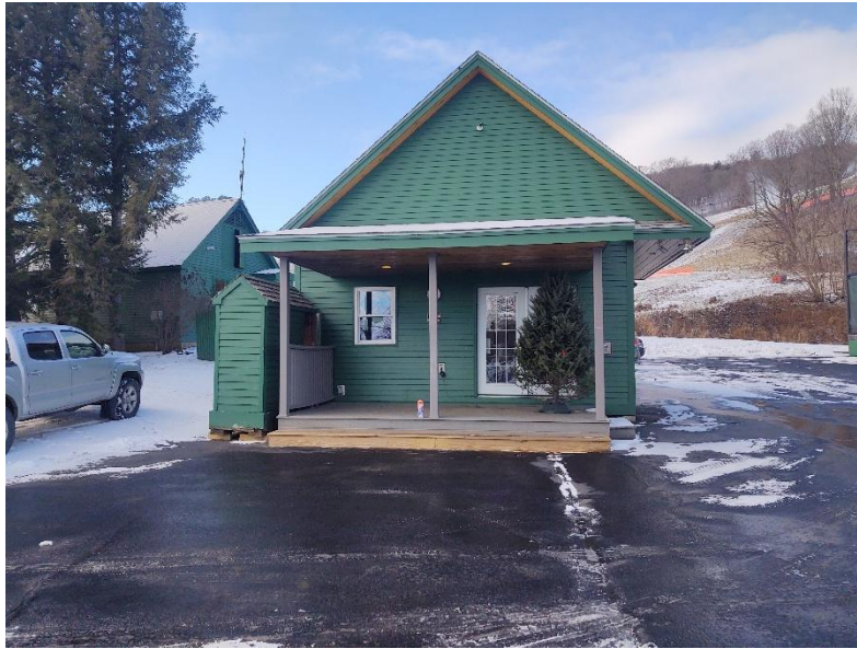
View of building to be removed.
